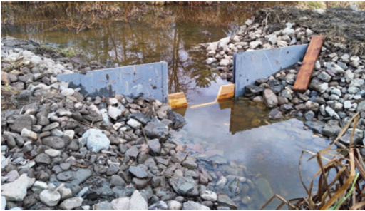
Photo 2. Spillway installed and first level control test using boards.
