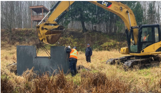
Photo 1. Plate to increase the water level just before installation.
